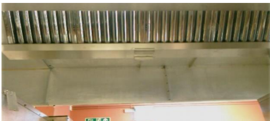
Underside view of retro-fitted replacement stainless steel filter housing incorporating stainless steel grease baffle filters and removable grease collection cups
