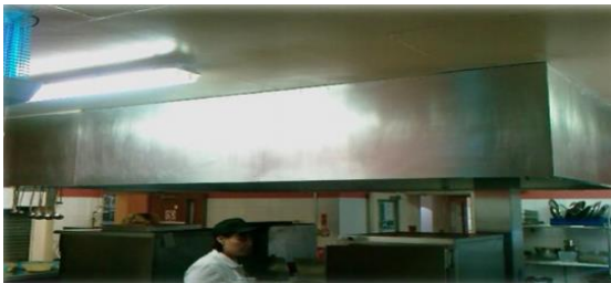
Existing canopy: Fit for purpose but does not meet new criteria
